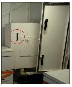
Figure 12: Picture showing the hydraulic oil tank outside storage room prior to the fire. Sight glass in the red circle.
